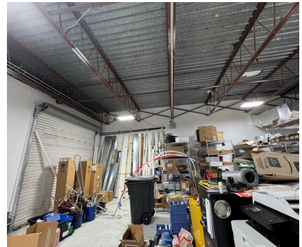
TWO SEPARATE WAREHOUSE SPACES
