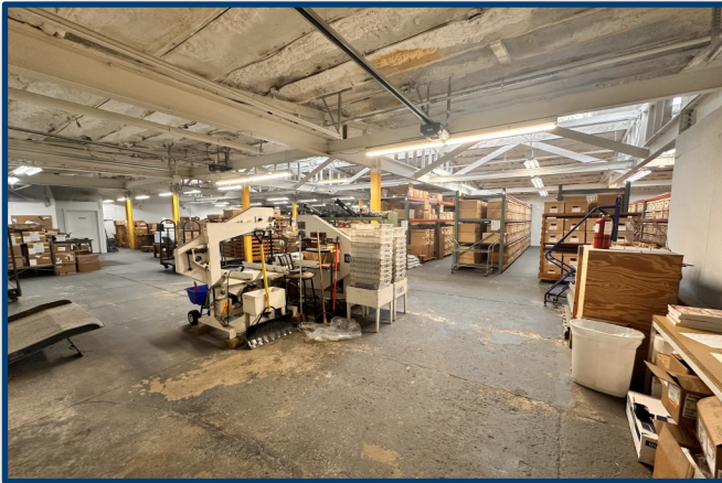
Warehouse Production Area
