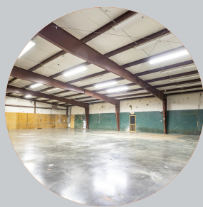
Clear span warehouse
