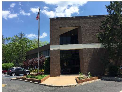
Building front main entrance
