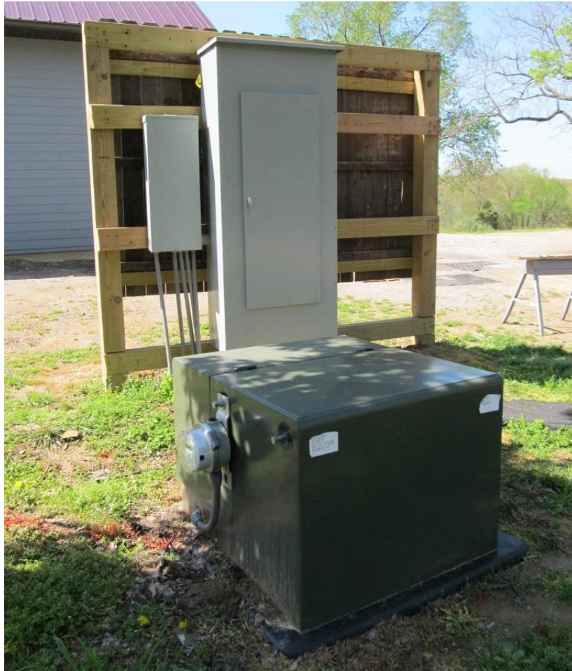
The main winery 25K amp transformer, 1200 amp powerboard and 200 amp outside service.
