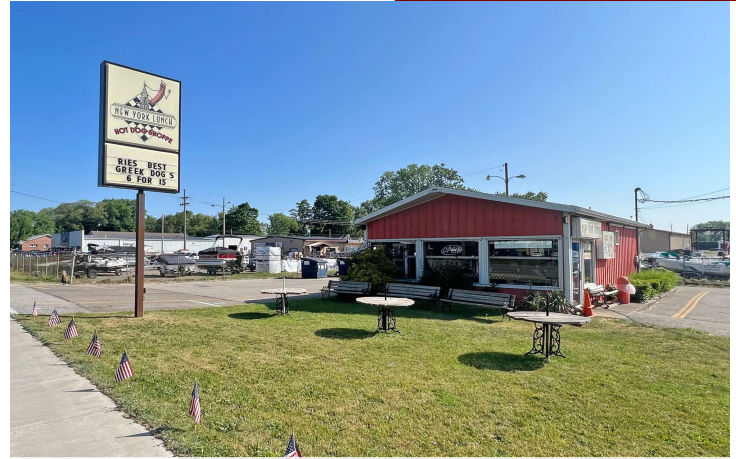
864± SF Restaurant with Drive-Thru at Signalized Intersection
