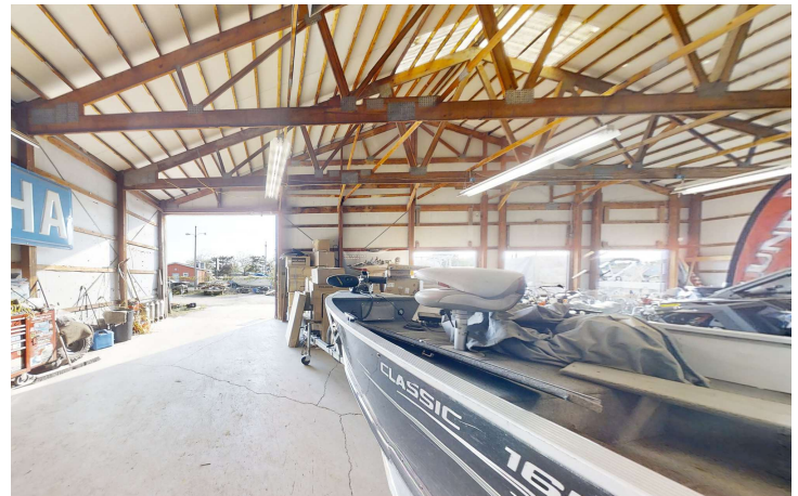
Building 2: 5,400± SF Warehouse
