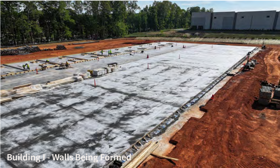
Building I - Walls Being Formed
