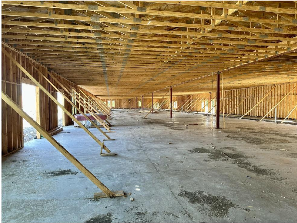
Interior - Shell Condition
