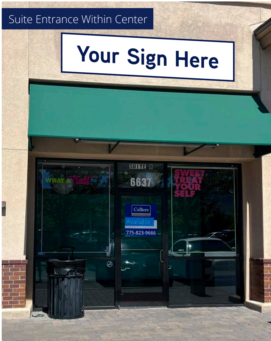
South Virginia Street View
