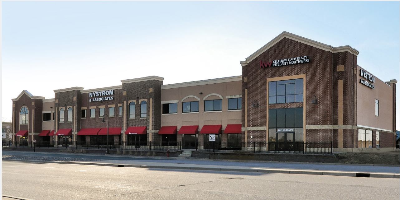
Front of Building
