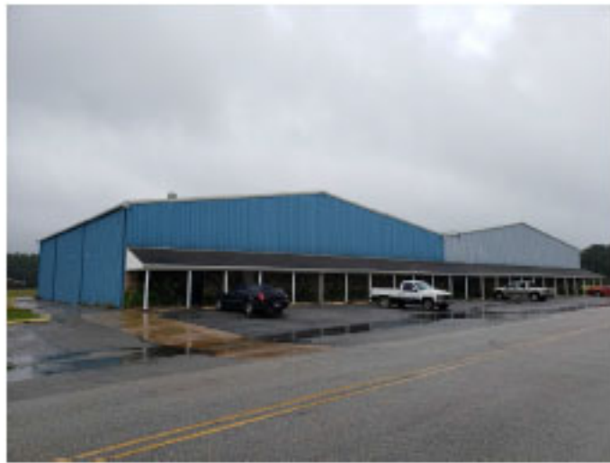
Exterior Building View
