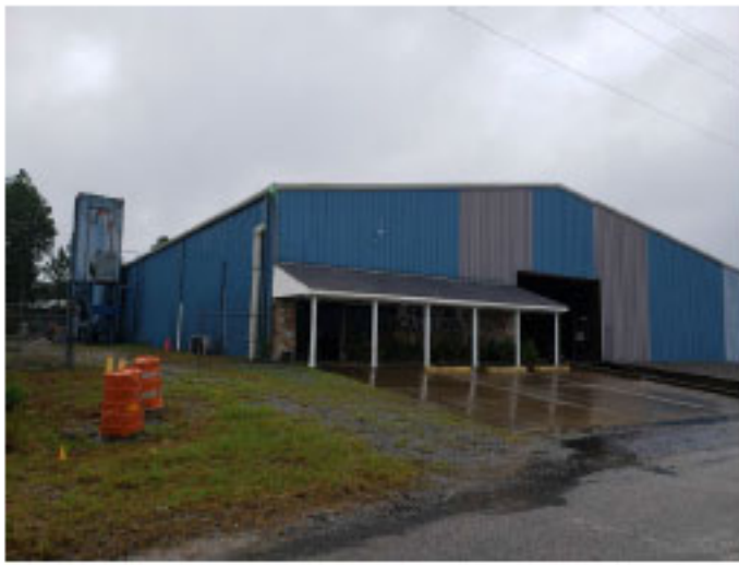
Exterior Building View
