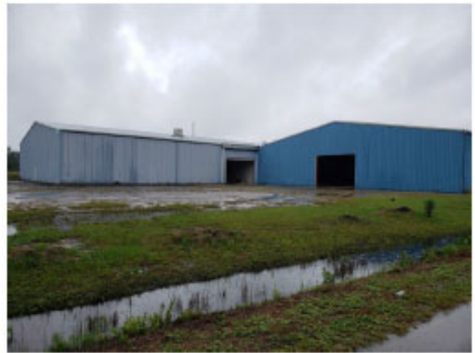
Exterior Building View
