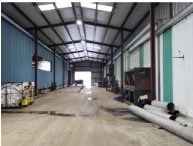
Interior Warehouse View
