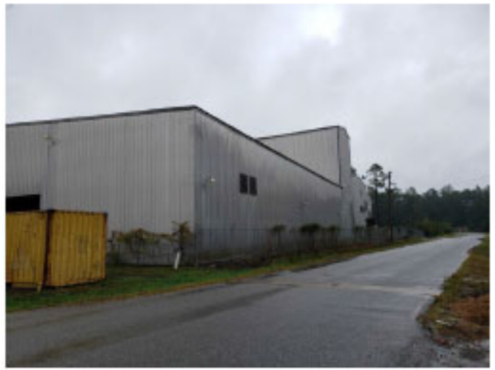
Exterior Building View
