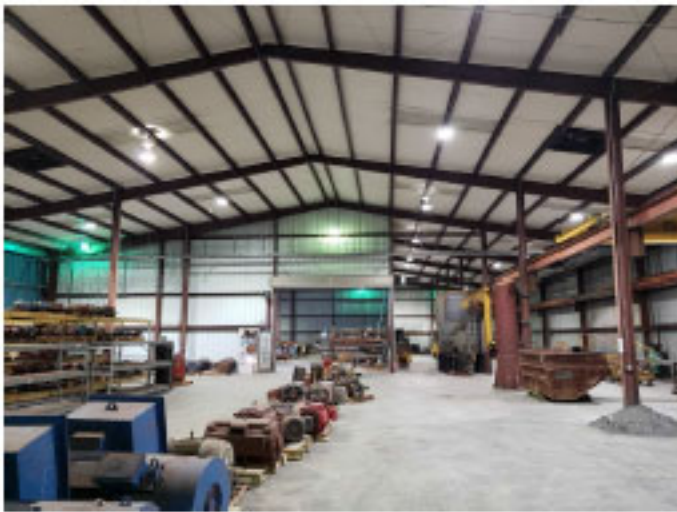
Interior Warehouse View
