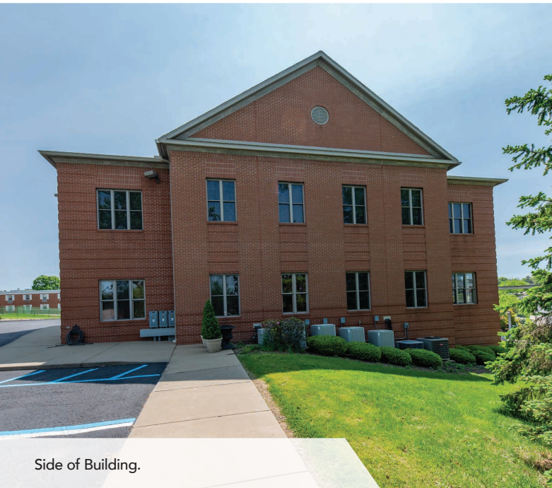
Back of Building/Parking Lot.
