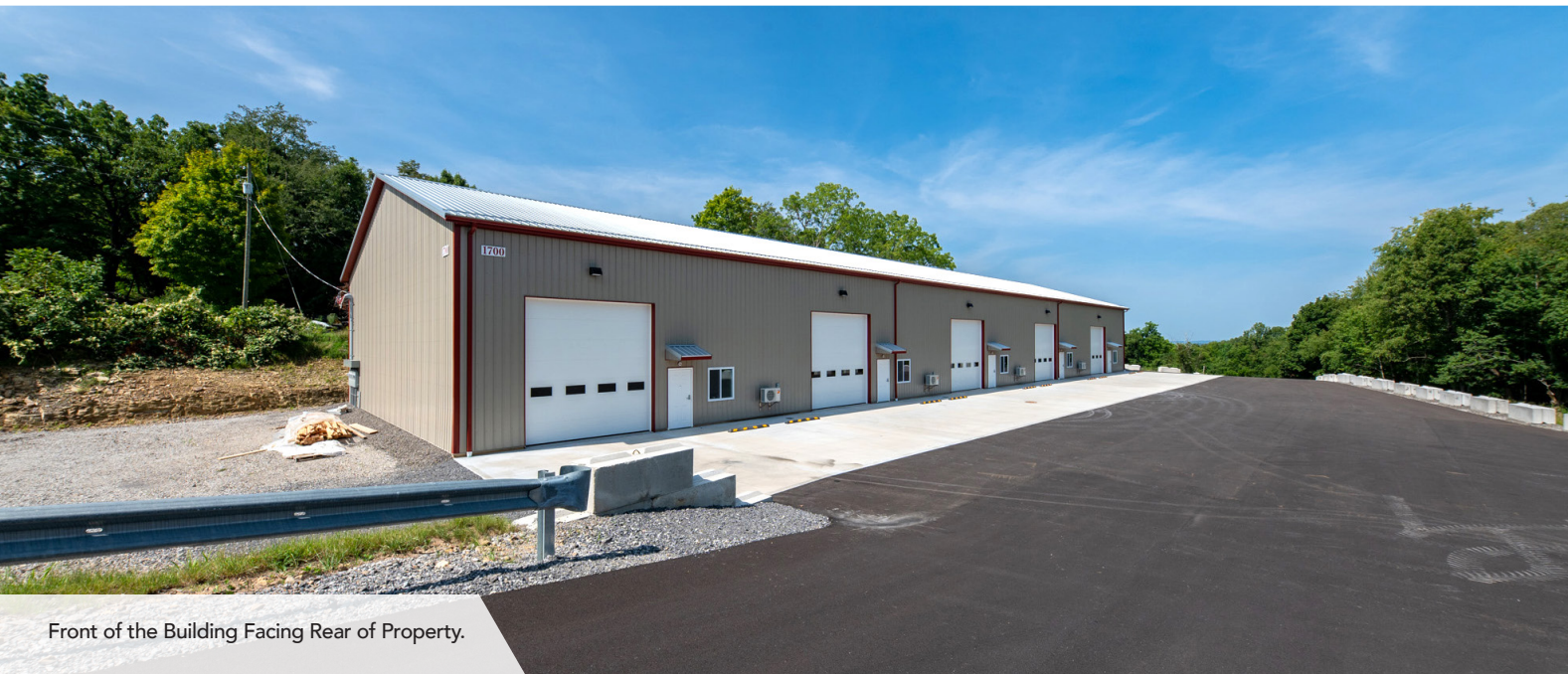
Front of the Building Facing Grafton Road.
