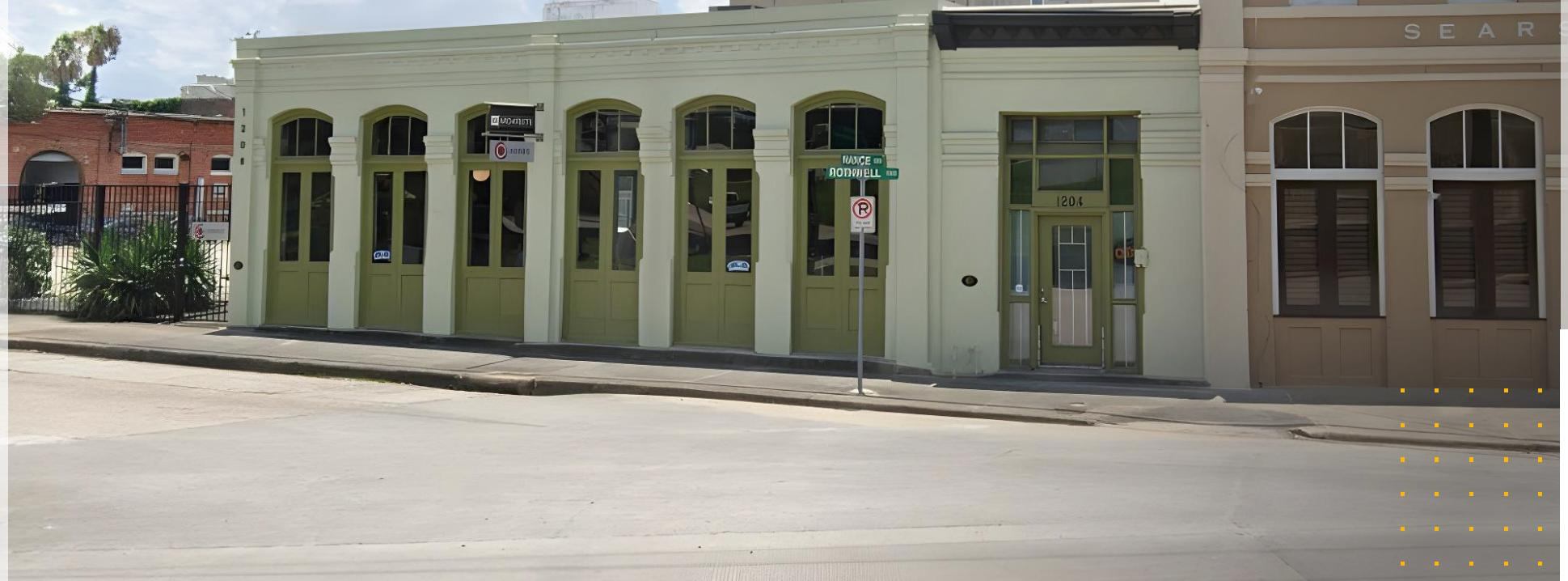
This former Fifth Ward Hotel is a rare survivor of Victorian commercial architecture in Houston. Completed in 1882, the building originally featured load-bearing masonry walls, cast-iron columns, and timber-framed floors. In 2002, the building's exterior was sensitively rehabilitated, resulting in a local Historic Landmark designation.
