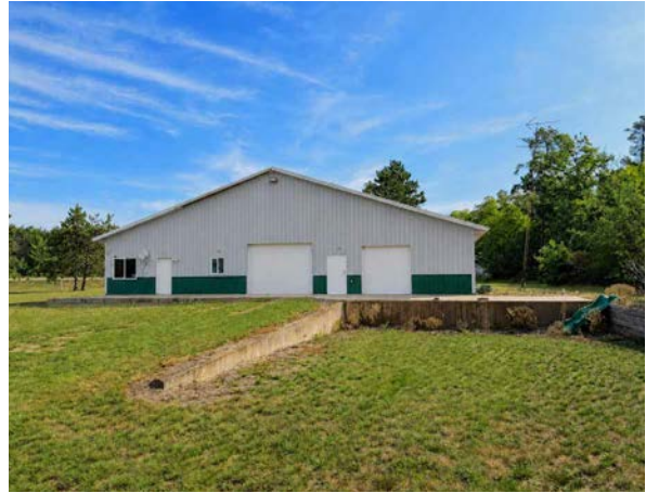
Overhead Doors & Loading Dock
