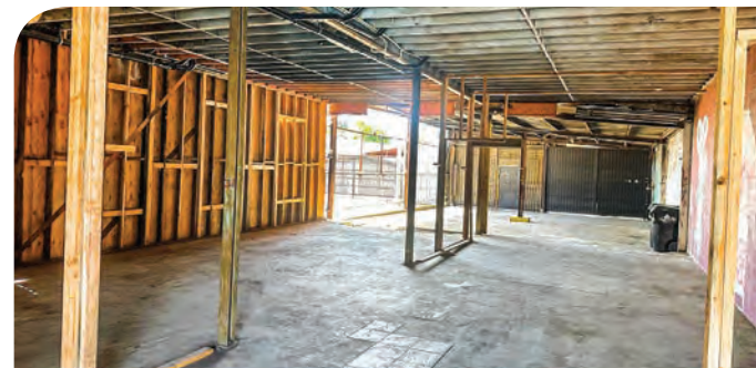
1424 W Slauson Ave - Interior View
