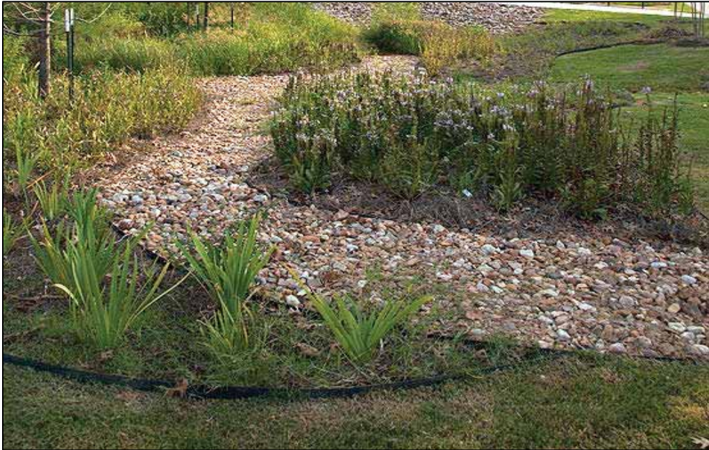
Figure 5.54. A combination of gravel to emulate the pattern of a natural creek bed and native materials help manage stormwater runoff while also improving aesthetic quality.
