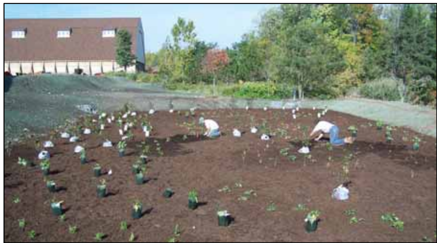
Figures 5.55 - 5.56. The Town of Penfield has a rain garden located along Jackson Road that provides a good example of how to sustainably address stormwater runoff. These images show a new planting (top) and the same garden after several years (bottom).
