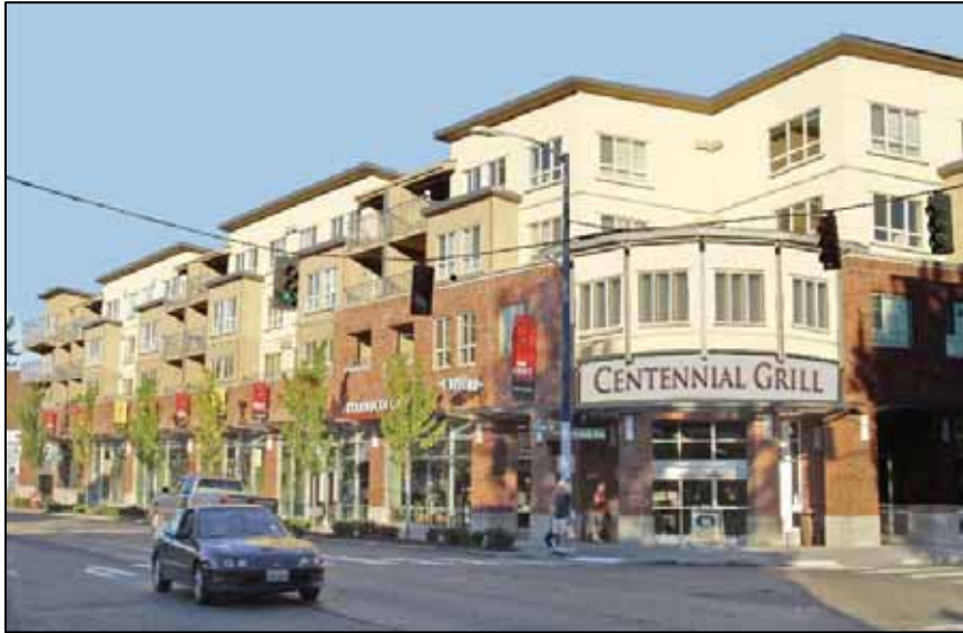
Figures 6.5 - 6.9. Vertical mixed use structures allow an increase in density while preserving space for pedestrian oriented activities. The lower level of vertical mixed use buildings should be commercial/retail services, while the upper levels should be predominantly residential (top, middle row). Residential uses (bottom) help provide housing within walking distance of commercial/retail mixed uses.
