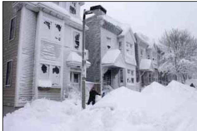
Figure 5.19 - 5.20. Street layout has to take into account snow removal, snow storage, and alternative routes in case one street or neighborhood is snowed in (below, top). This street layout plan (below, bottom) shows the type of interconnected streets, lot layout, and integrated open space that helps make mixed use developments more walkable communities.
