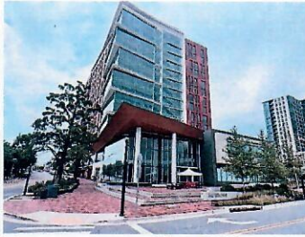
New county office bldg. Directly across the street
