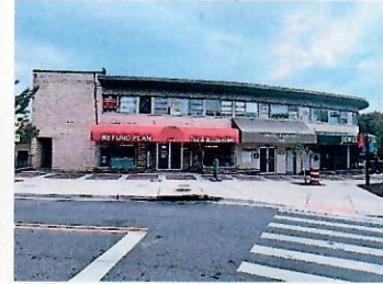
Exterior of building
