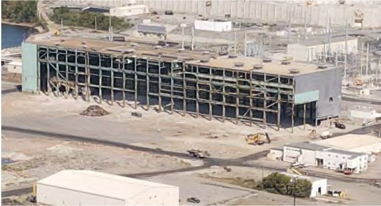
Ideal Mfg. Bldg. (630' x 130') features 100' ceilings & two 100-ton cranes
