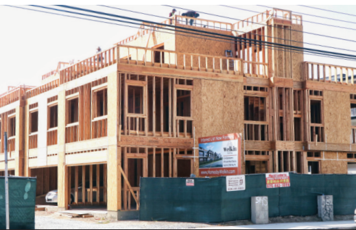
New homes across the street
