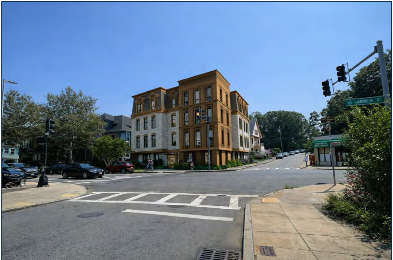
Existing and as approved with 556 Cambridge Street front and center
