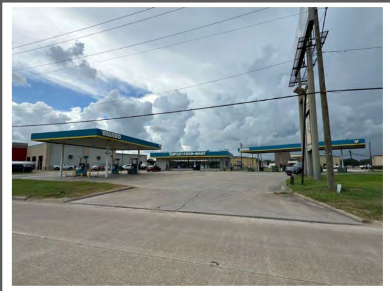
Site view across W. Cardinal Drive
