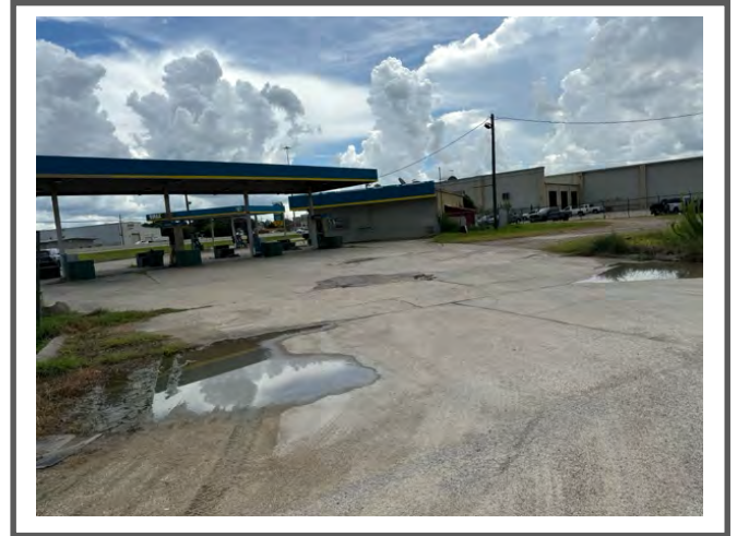
Site view across Gorman Road
