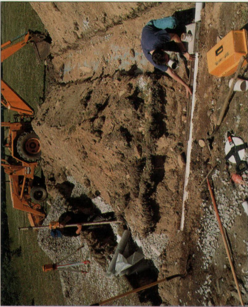
Conventional stone and pipe system
