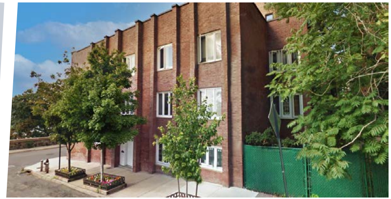
View from West 186th Street of garden fence.
