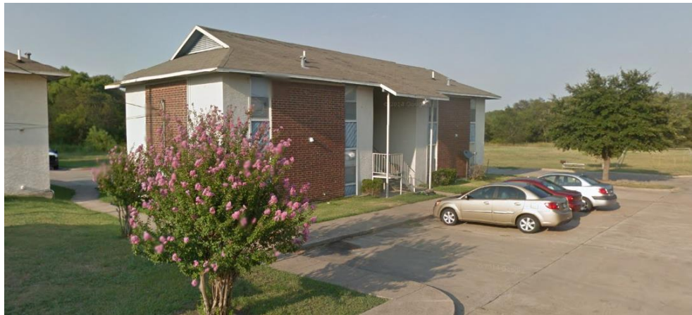
Undesirable - Inadequate Front Facade and Roof Articulation
