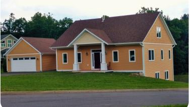
performance.Our windows -triple-paned, inert gas filled, low-E -exceed Energy Star performance criteria by at least 30%.Finally, we use twice the insulation required by Energy Star beneath the slab (4 inches total rigid insulation providing R-20) to complete our ground-to-roof, energy efficient thermal envelope.
