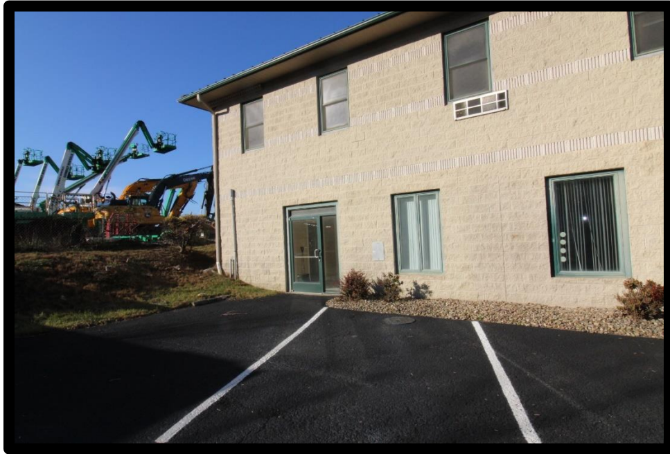
REAR OUTSIDE ENTRANCE TO LOWER-LEVEL STORAGE-OFFICE
