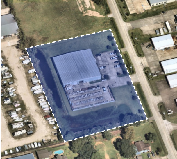
1860 Lawrence Rd Great Western Valve
