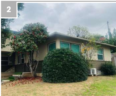
2 7030 RAMSGATE AVENUE Los Angeles, CA 90045
