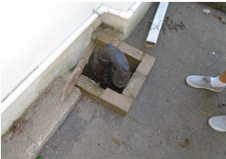
Disconnected pipe
