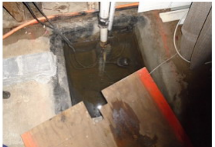
Sump pit - no obvious concern
