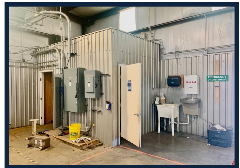
ADA Restroom and Closet
