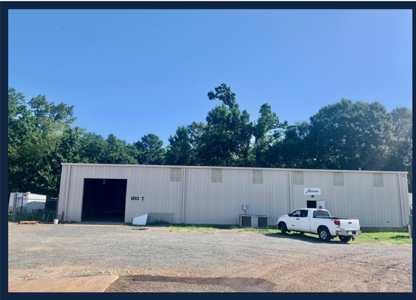
Front Overhead Door Access
