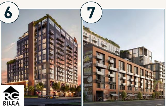
N.E. 29th St The Rider and Mohawk Wynwood Under Active Construction
