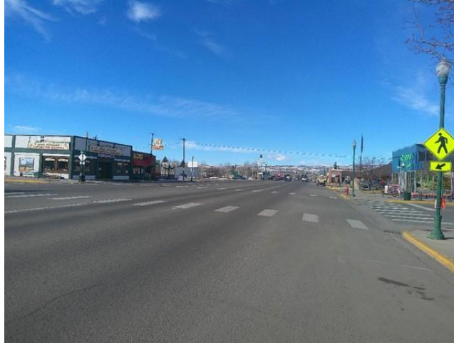
W. TOMICHI AVENUE FACING WEST - SUBJECT TO RIGHT
