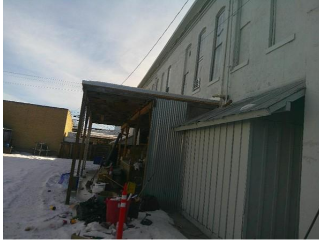
NORTHERN SIDE OF SUBJECT
