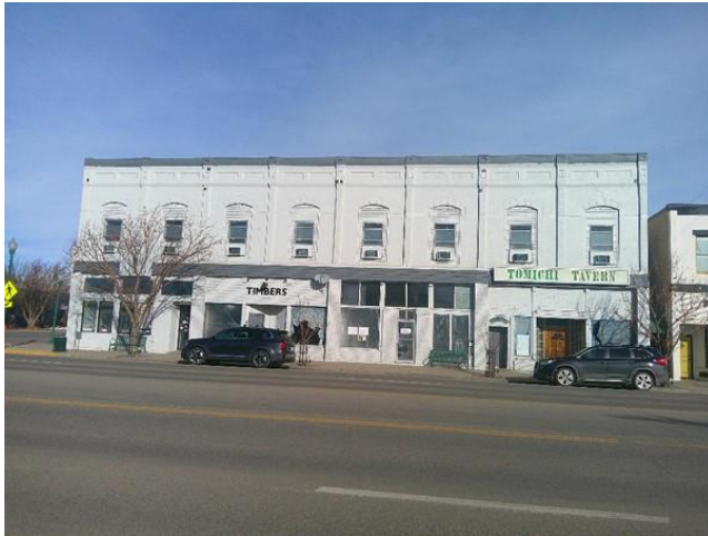
FRONT OF SUBJECT ALONG TOMICHI AVENUE
