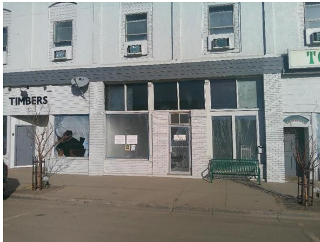
FRONT OF MIDDLE UNIT
