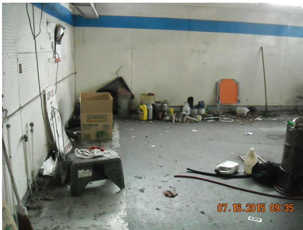
PHOTO 10: Auto repair fluids and materials left behind by former tenant
