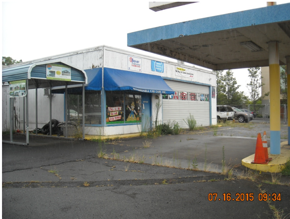
PHOTO 1: Looking northeast toward the former auto repair structure
