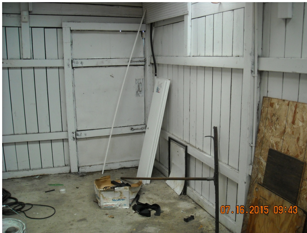
PHOTO 12: Storage shed located at the northwest corner of the structure (attached to building)
