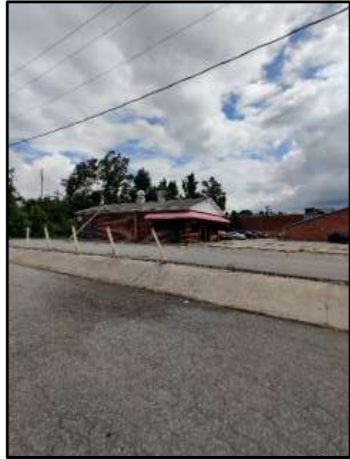
Adjacent buildings, West
