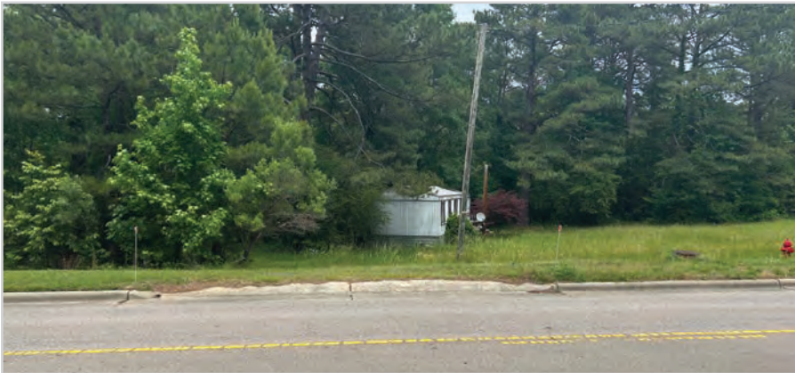
Curb Cut/Driveway at 5814 Smithfield Rd
