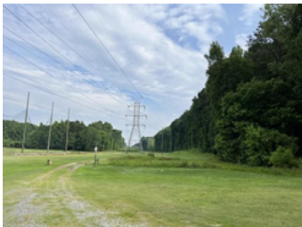
TYPICAL VIEW OF REAR EASEMENT AREA
