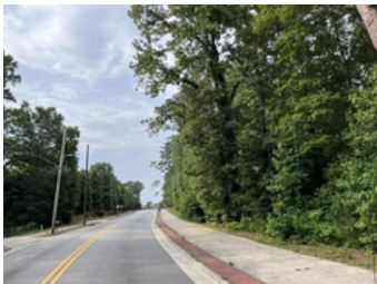
NORTH ALONGFAIRBURN ROAD, SUBJECT AT RIGHT
