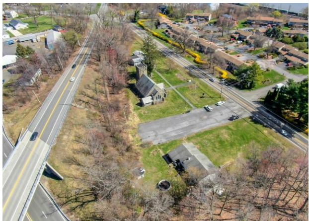
Aerial -- Campus, Parking Lot & Route 9W Corridor
