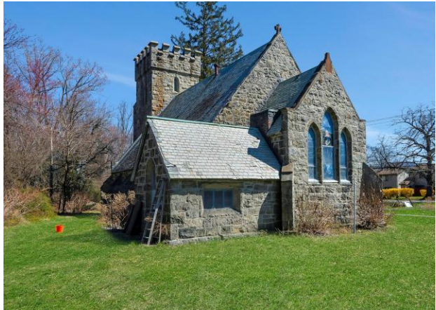
Church Rear Elevation & Slate Roof Detail
