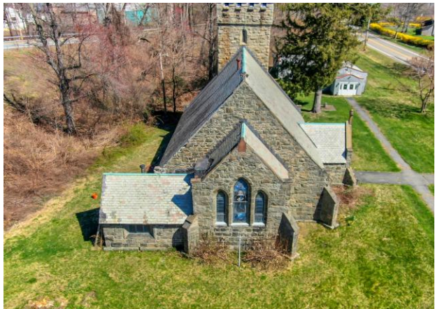
Aerial -- Church Campus Looking North
