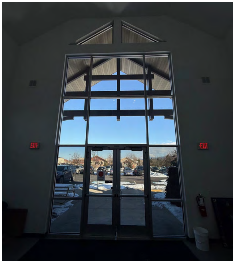
East End Entrance
