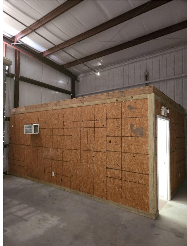
610A Insulated roof, office space
