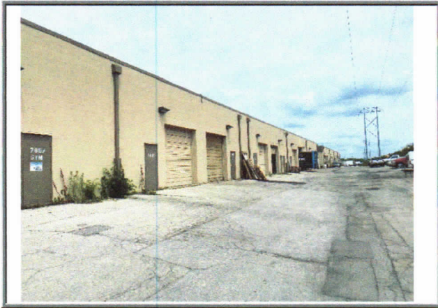
East side of both buildings looking north
