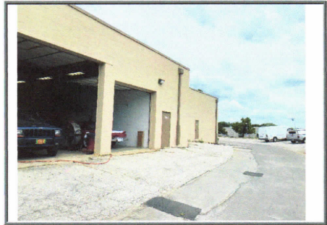
East of the north building looking north
