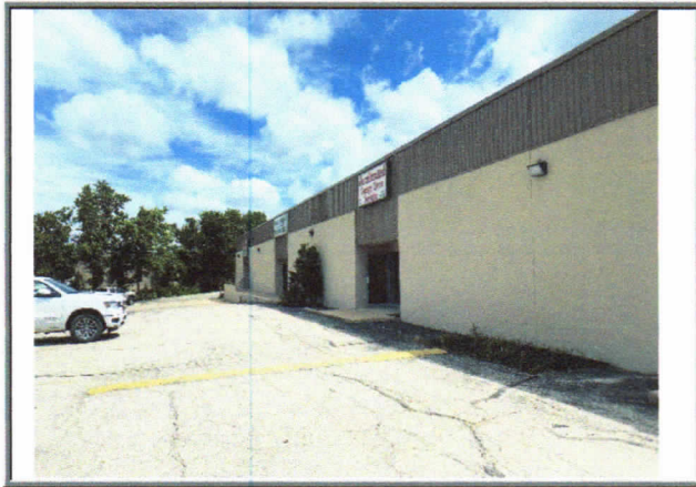
West side of north building looking north
