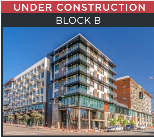
Broadstone Makers Quarter • Delivery Q2 2018 • Seven stories with 269 residential units • ±5,015 SF of retail with Broadway Frontage
