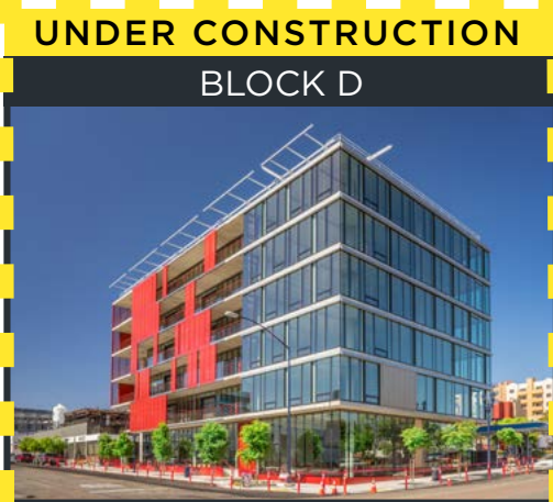
Block D • Under construction / delivery Q2 2018 • ~45,000 SF of creative office • ±4,553 SF of retail / restaurant
