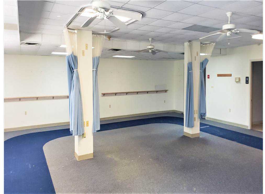
Rehab interior track
