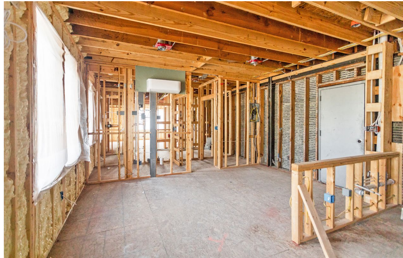
Typical Kitchen & Living Room
