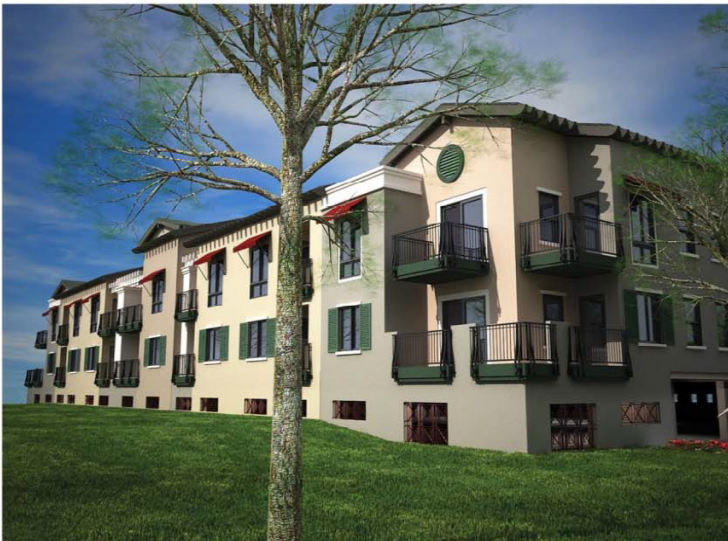
Podium Building From Street Corner
