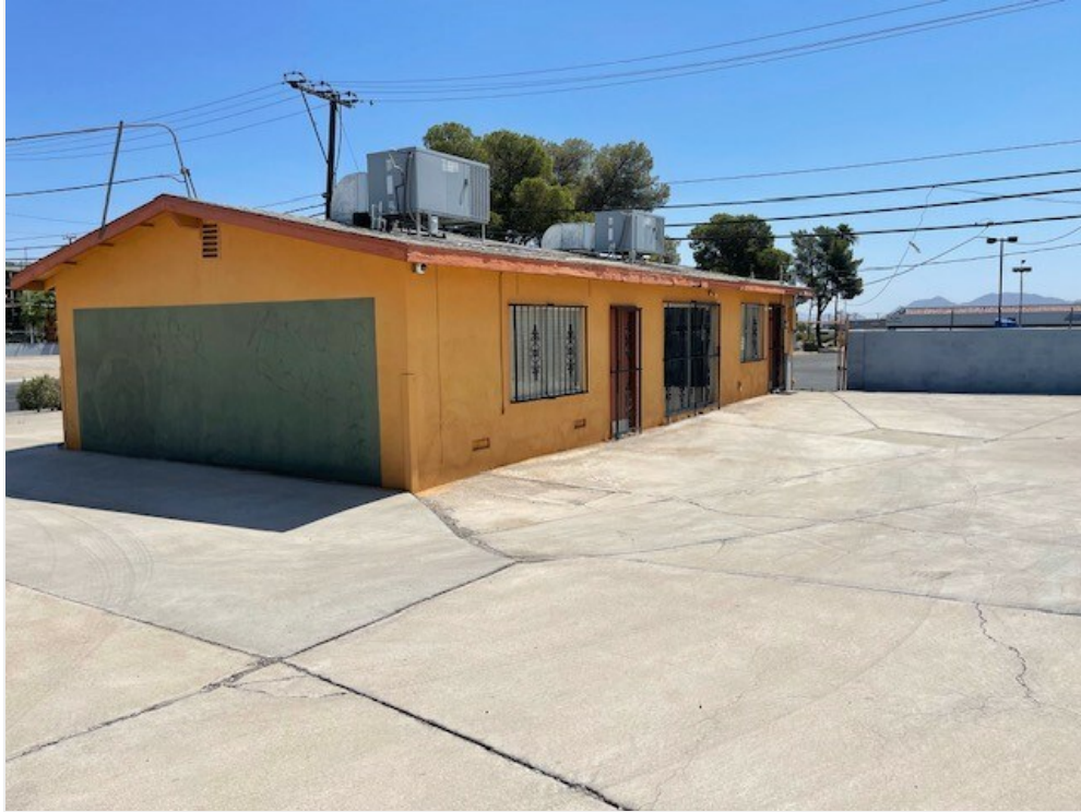
5017 Rear Building View
