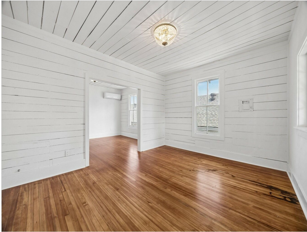
46 Two large flex rooms feature shiplap walls and red oak floors all original to the house and refinished.
