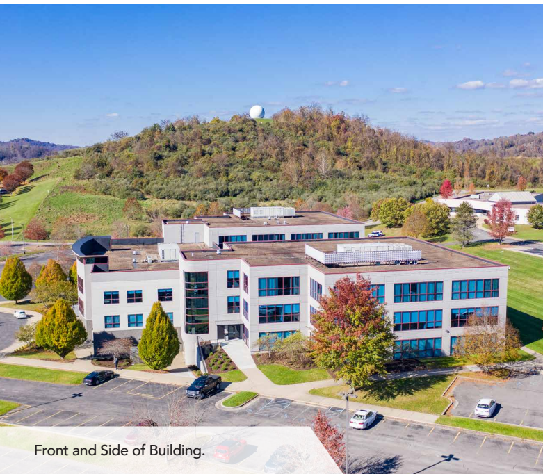
Front of Building.
