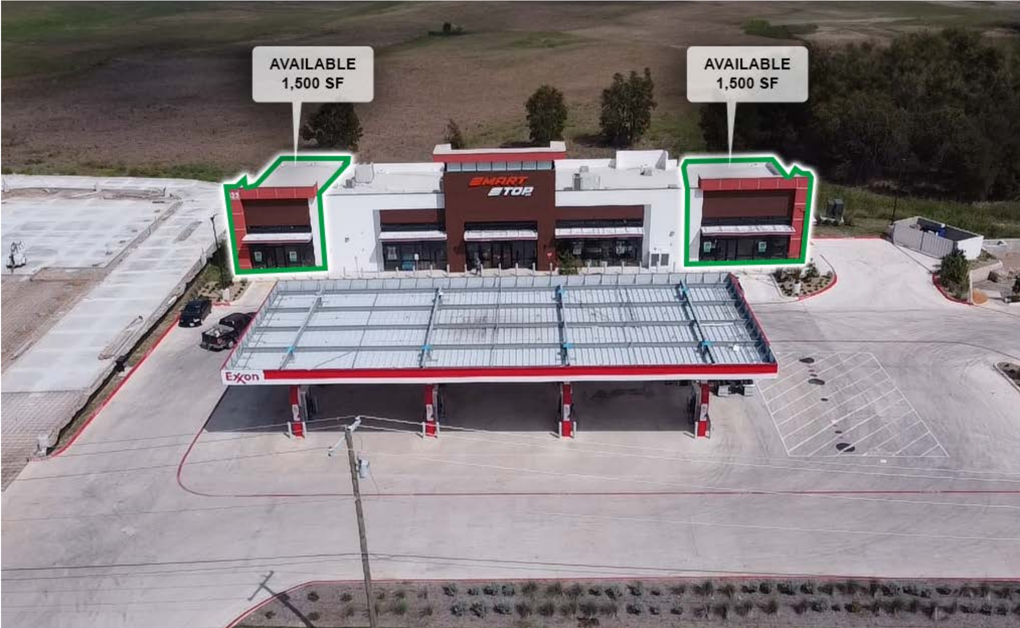
Construction Progress Aug 2024
