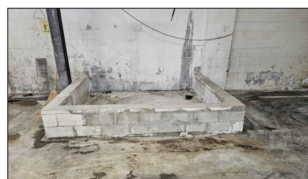
24 A2 INTERIOR VIEW
